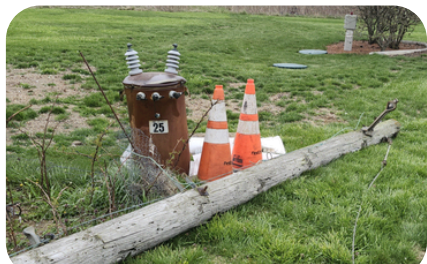
Fallen utility pole with release of Non-PCB transformer oil into nearby drain
